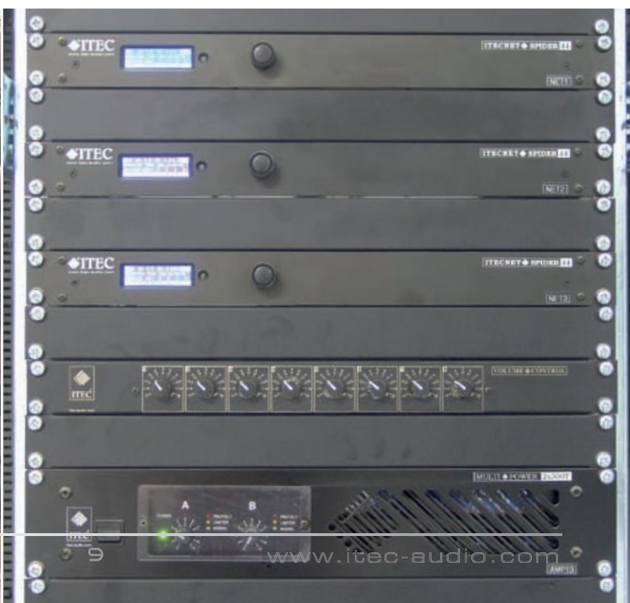
One of the numerous racks with "Spider 44" systems and power amplifiers – On the right 3 "Spider 44" systems with level regulators as mentioned within the report
